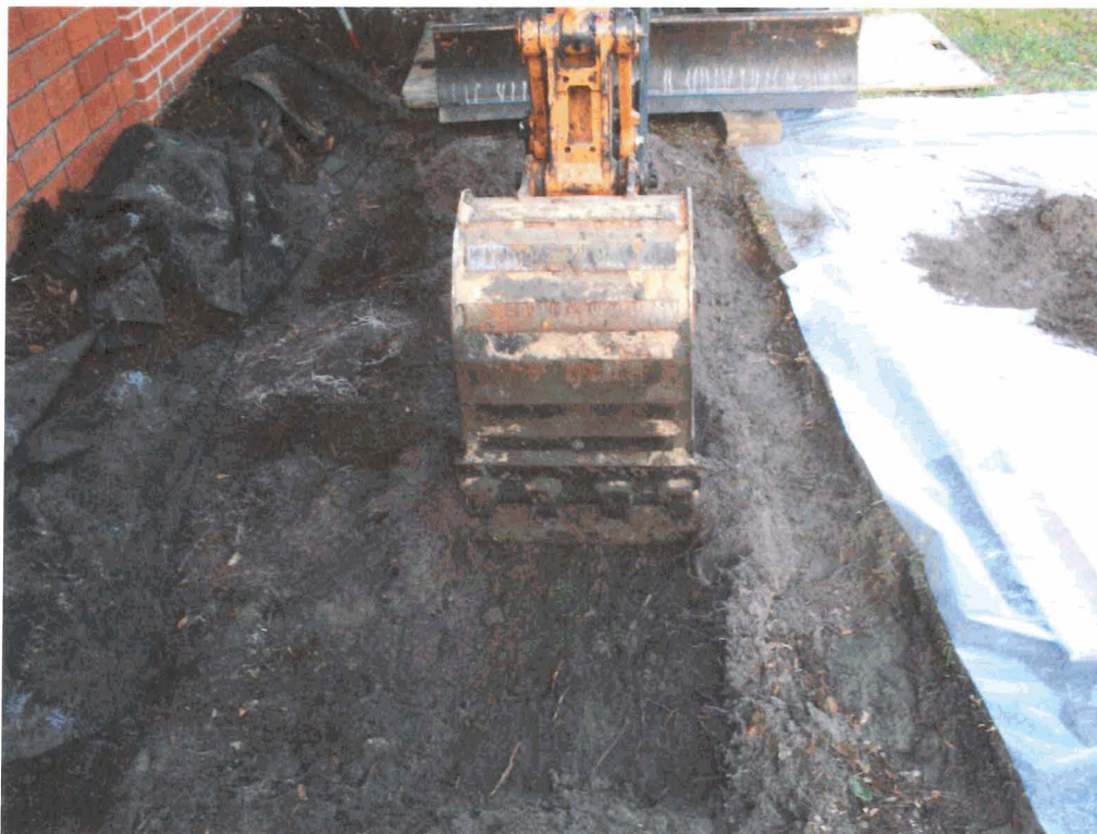
Picture 2: UST 1302Eagle excavation in progress.
